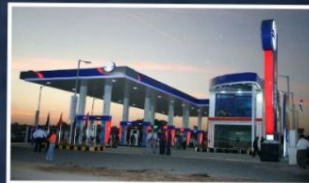
HP Petrol Pump - Mumbai Pune Highway
