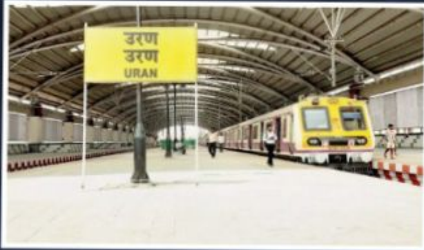
Railway Project - Uran
